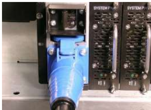
Figure 10-2 Attaching the power cord
