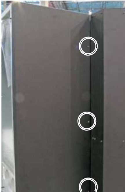
Figure 6-16 Installing the side panel on the expansion pod
