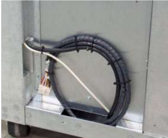
Figure 6-4 Expansion-pod controller cable on the side of the XLS-812300
