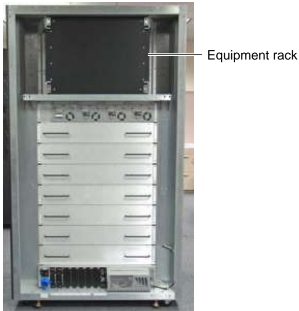
Figure 7-1 Back of XLS-832700 with the optional equipment rack installed
