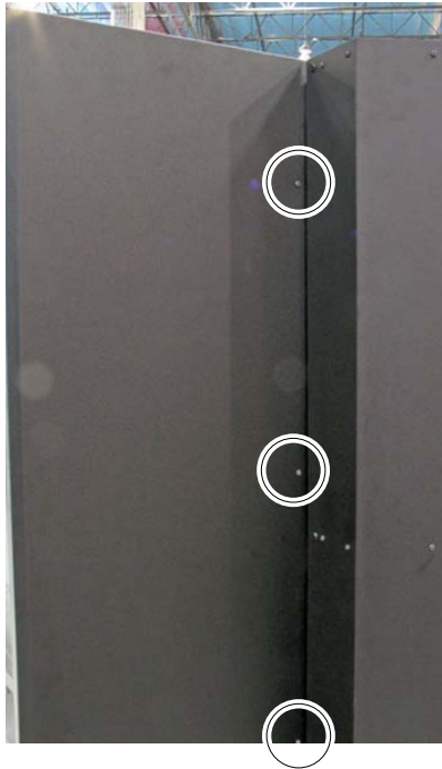
Figure 6-15 Installing the side panel on the expansion pod
