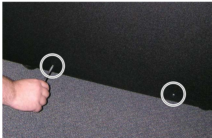
Figure 5-15 Installing the side panel on the MEM
