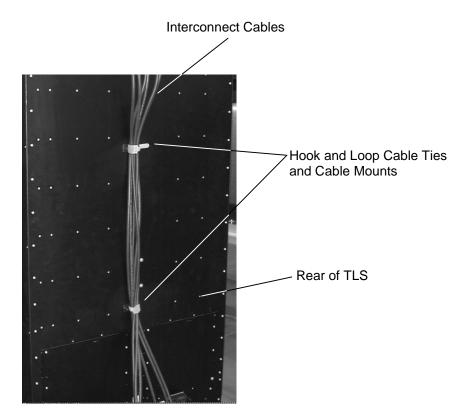
Figure 5-8 Example of Cables Secured to the Rear of the TLS
